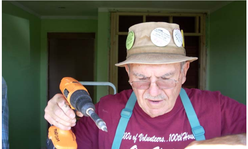
Virgil Horton works on the Joy St. rehab this past summer.
